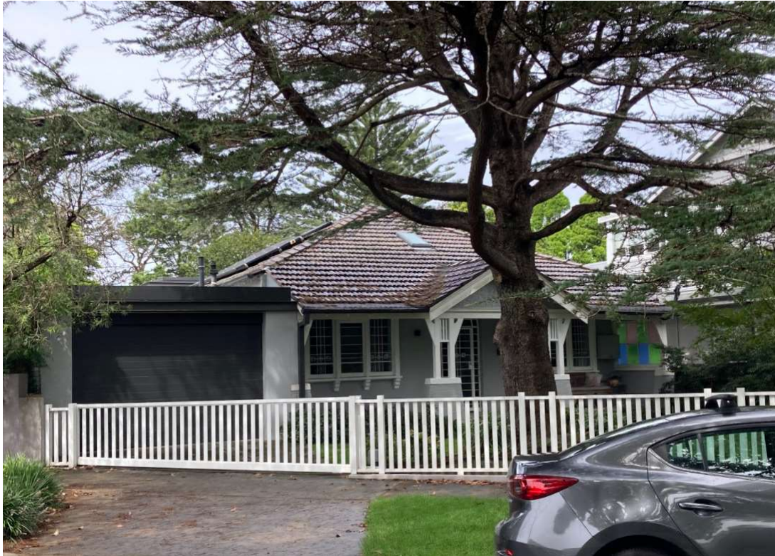
Figure 6: 15 Riddell Street, viewed from street frontage.
